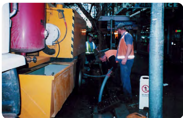
Photo 11 Cleaning an EnviroPod using the inductor method
