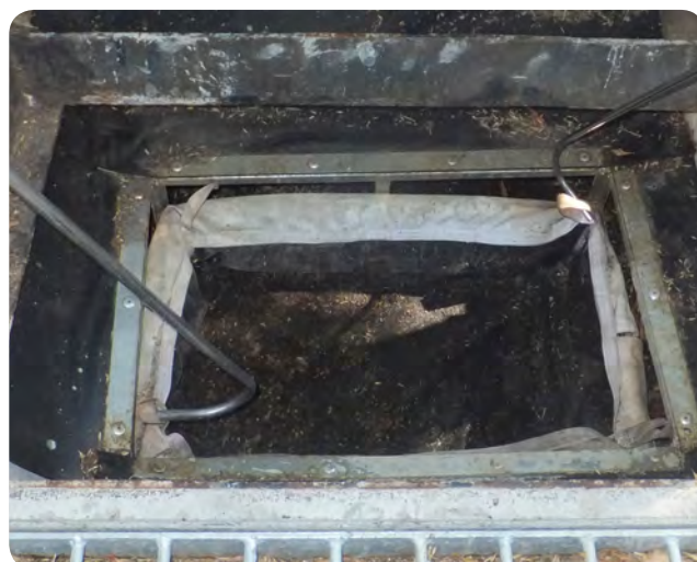
Photo 21 Correctly installed filter bag
