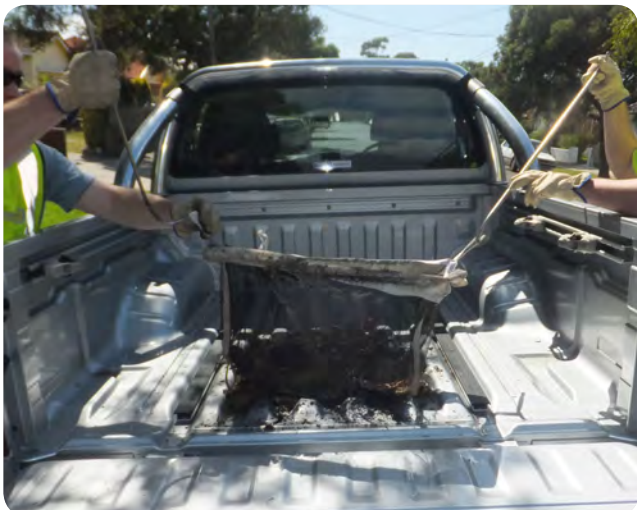
Photo 16 Grab the bottom lifting loops
