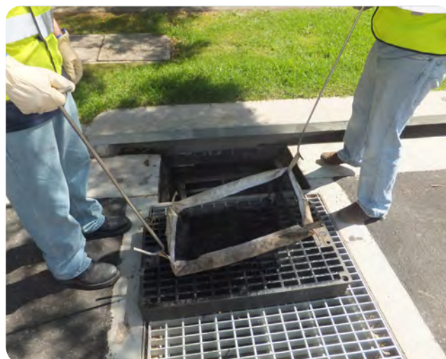
Photo 19 Reinstall filter bag
