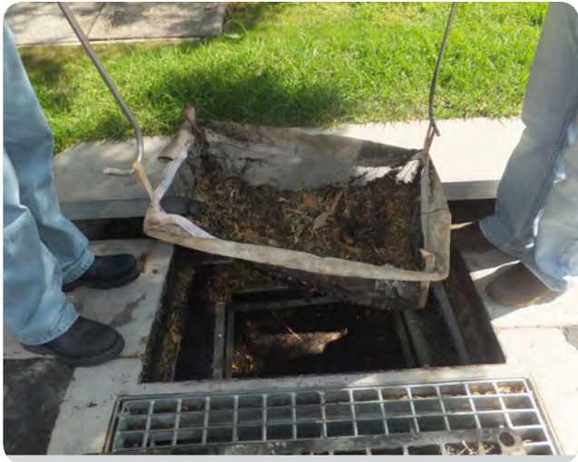
Photo 14 Lift the bag from the stormwater pit
