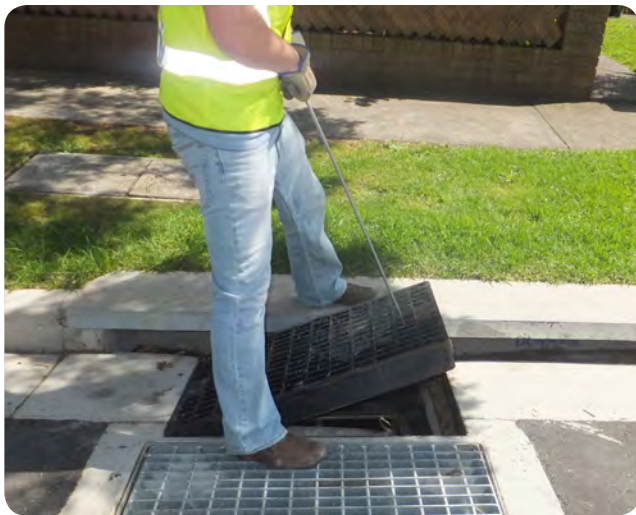
Photo 3 Lifting the grate
