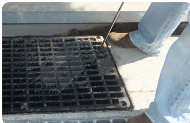
Photo 6 Insert hook near edge of grate
