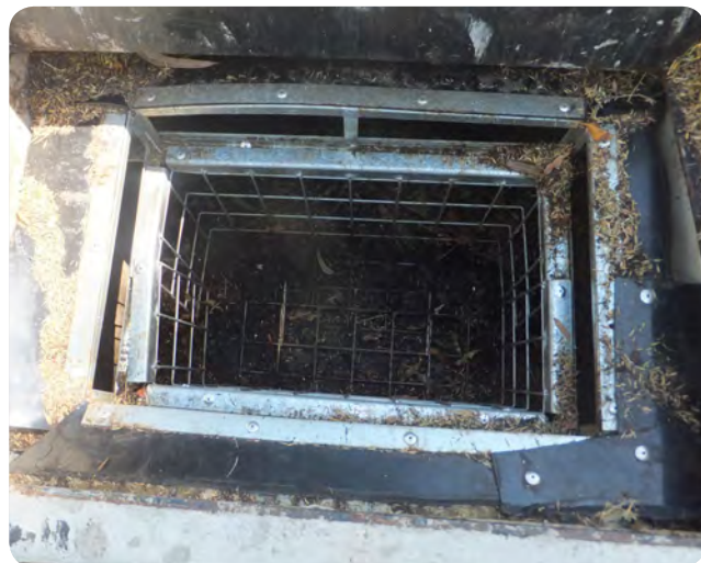
Photo 24 Check joining rivets (two piece unit shown above)
