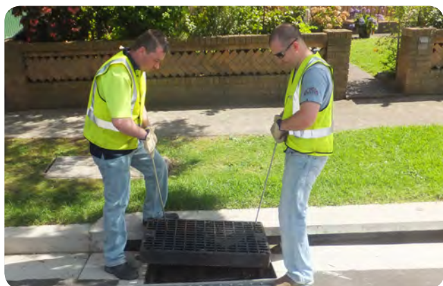
Photo 9 Lift grate above the support frame
